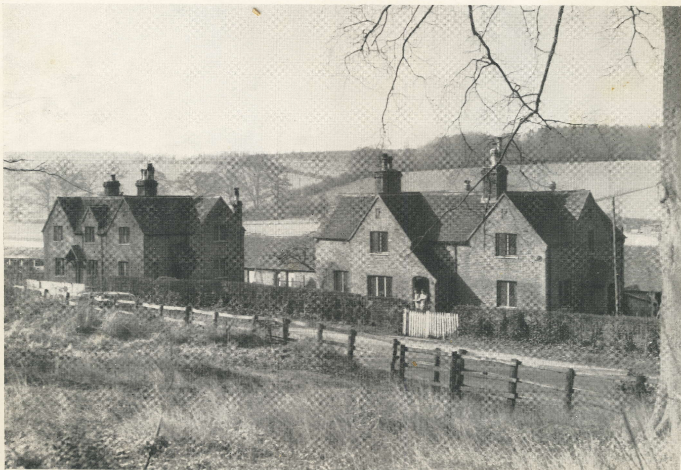
Nos. 2-7 CHESHAM ROAD
