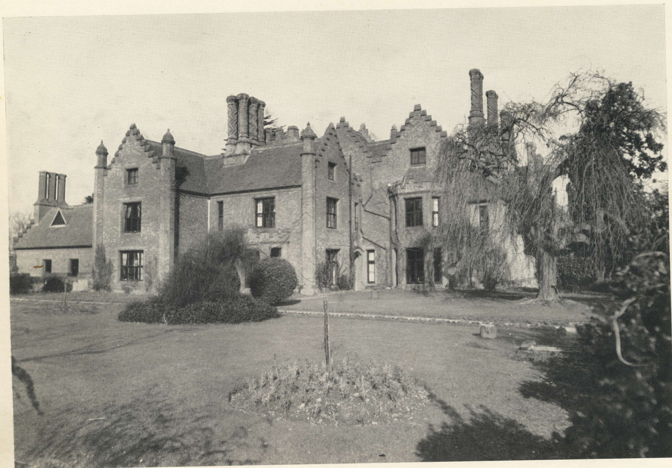
LOT 3. GREAT HOUSE FARM—THE HOUSE
