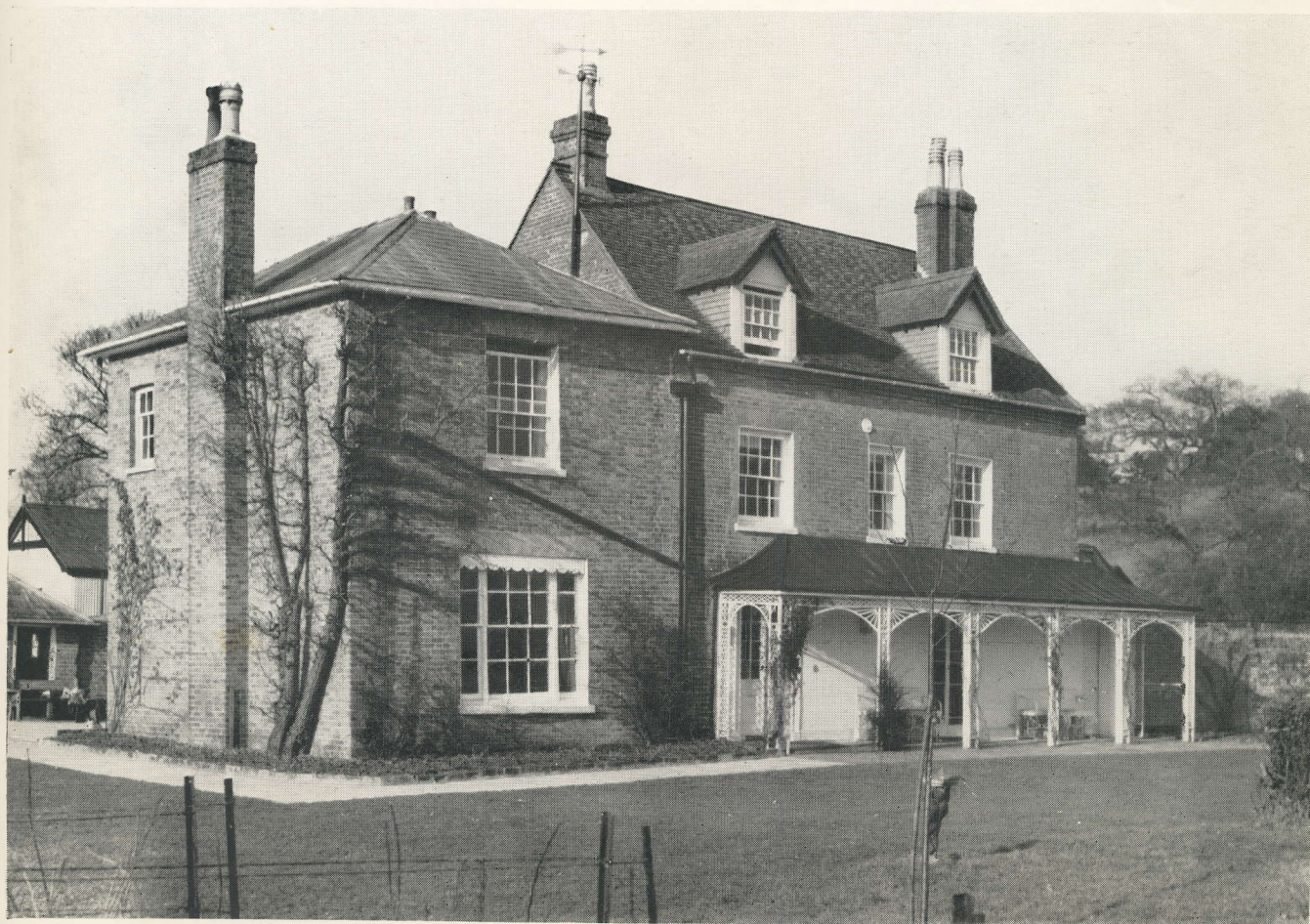
LOT 28. SABBATT MILL HOUSE
